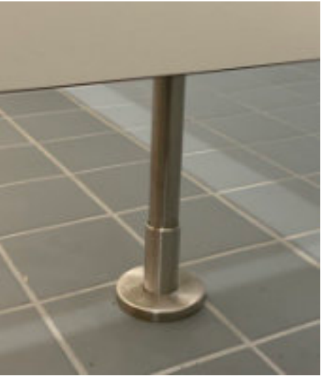
Pedestals made entirely of stainless steel 304
