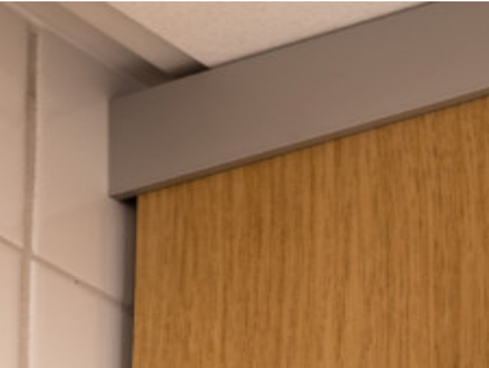
Wall connections via shadow gap made of satin anodized aluminum
