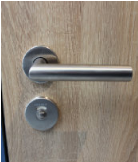
L-shaped door handle made of stainless steel
