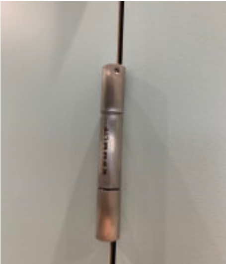
3-roller edge spring hinges made of stainless steel
