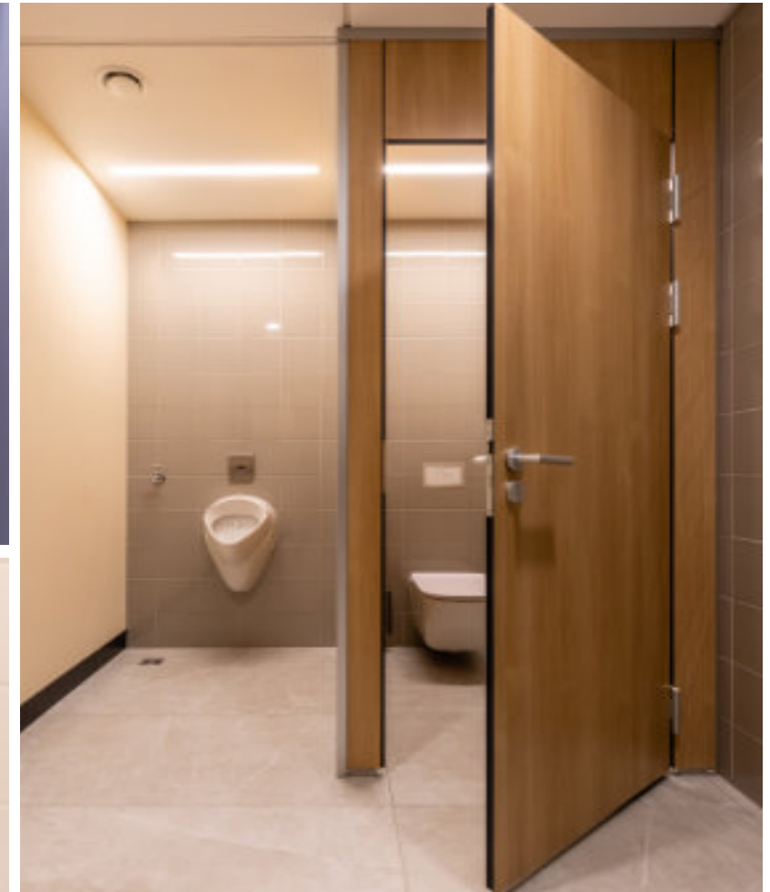
Configuration floor-to-ceiling with transom panel above the doors, L-shaped door handle in aluminum and wood decor
