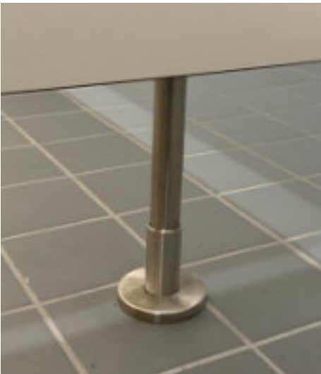
Pedestals made entirely of stainless steel
