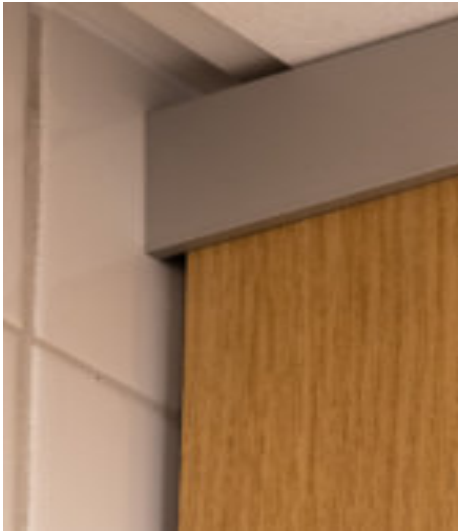
Wall connections via shadow gap made of satin anodized aluminum
